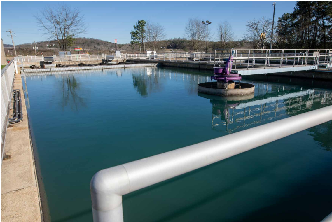
CARSON FILTER PLANT
