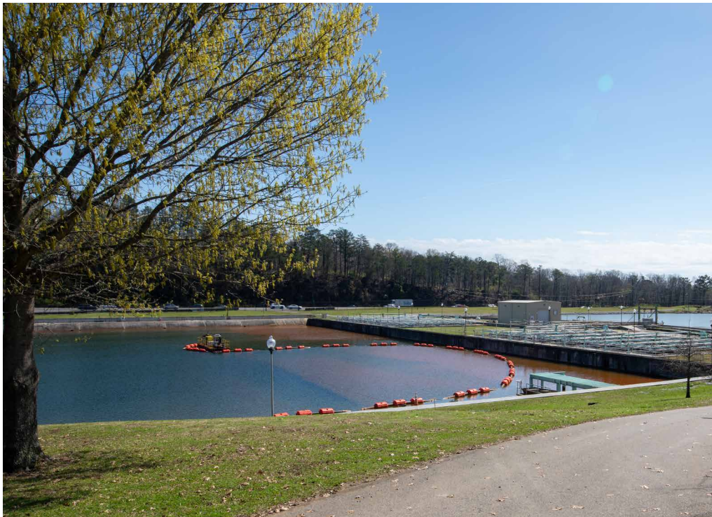
SHADES MOUNTAIN FILTER PLANT
