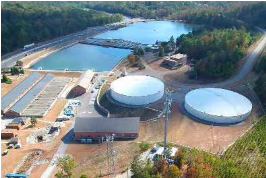
SHADES MOUNTAIN FILTER PLANT
