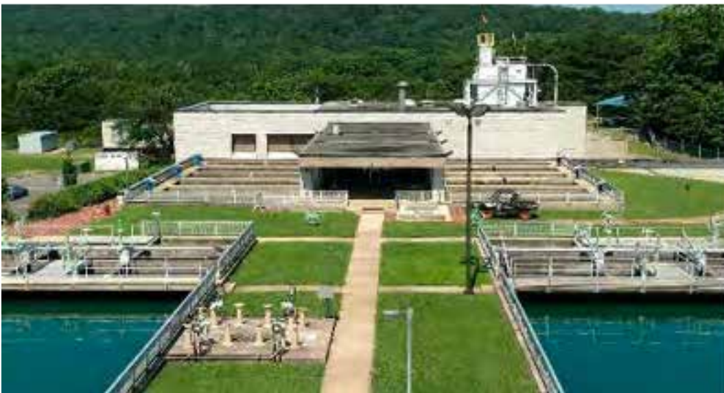
CARSON FILTER PLANT
