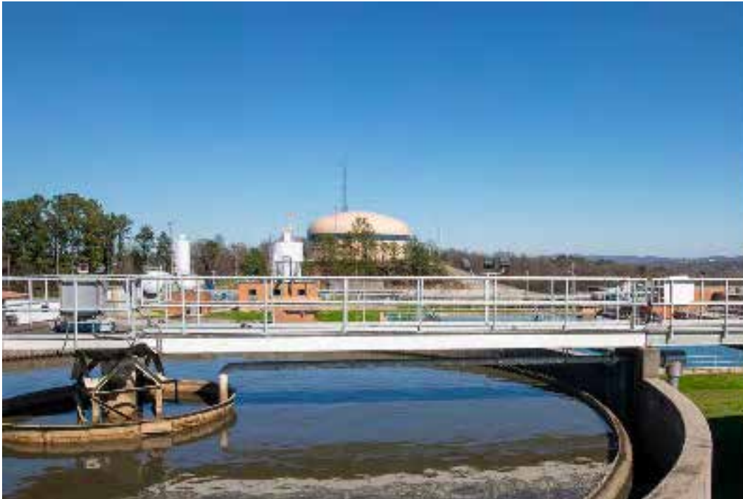
WESTERN FILTER PLANT
