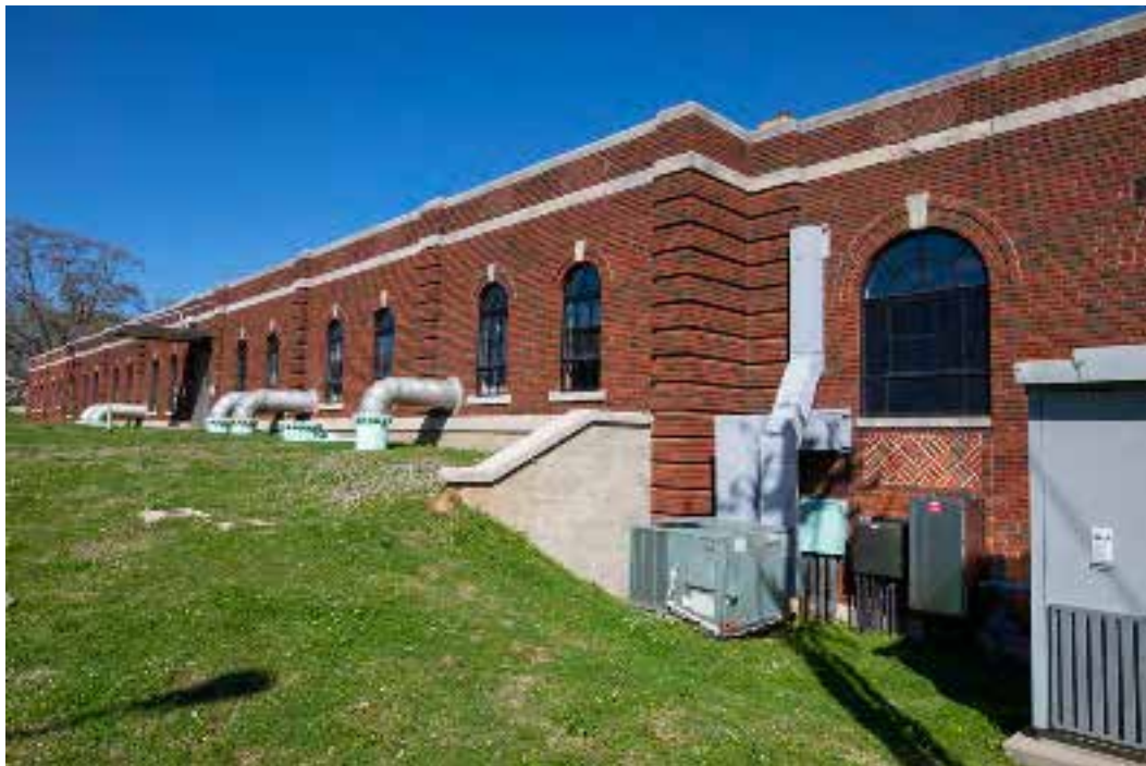
PUTNAM FILTER PLANT
