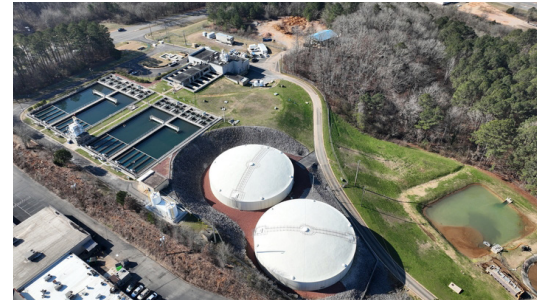
Pictured: Award-Winning Carson Filter Plant
